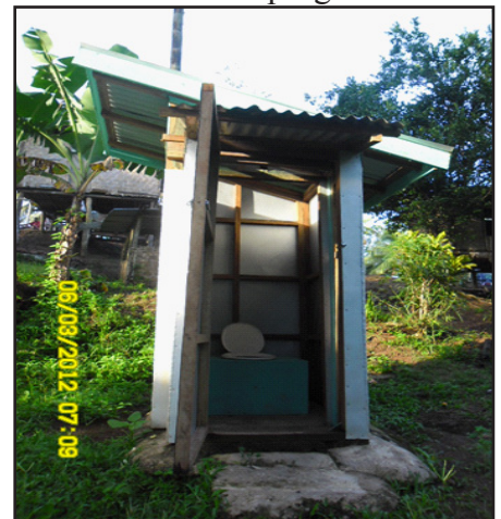
Ventilated Improved PIT LATRINES recently constructed, 2013.
