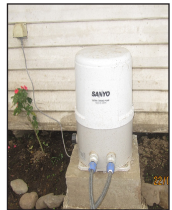
Above: Reserve Tuffa water tank installed at Anglicare MT.Hagen. Below: Sanyo electric water pump installed.
